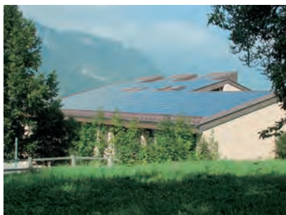
Left: 224 kW installation; on a total of 14 residential buildings in the Ruggächern development, in Zurich.
