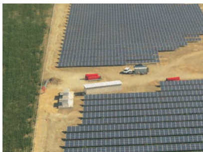
Left: The El Tesoro solar power plant with a 1 100 kW total installed capacity; of which 550 kW are owned by Edisun Power.
